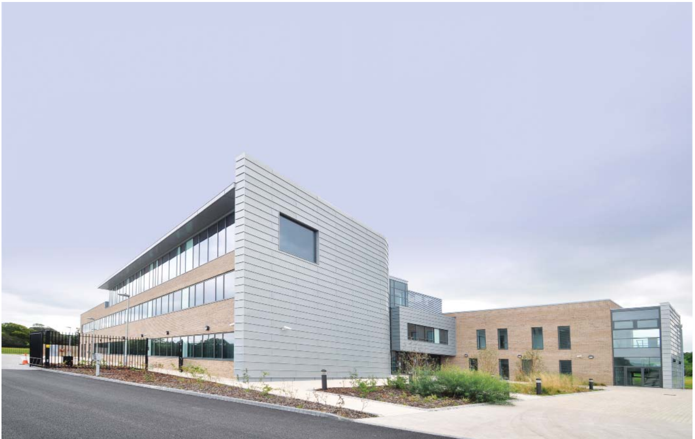
Photograph 1 – The Welsh Government and Dyfed Powys Police Force have built a new bespoke Strategic Coordination Centre in Carmarthen, one of three such centres in Wales.
